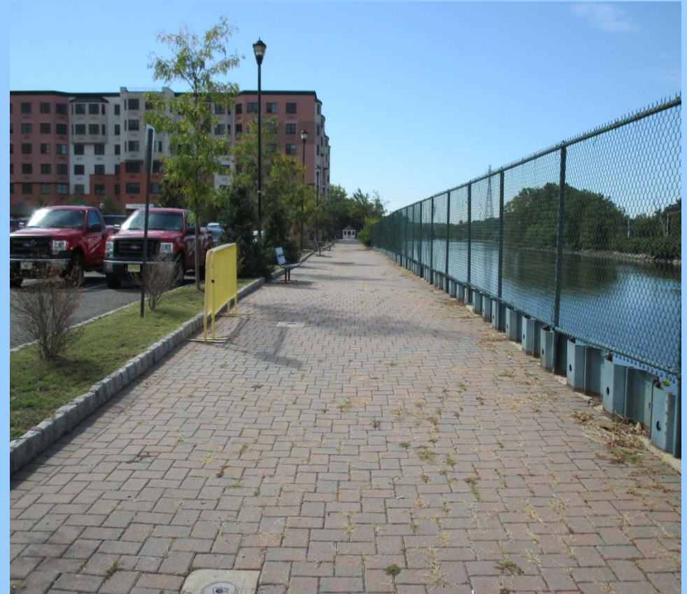
Passaic River Waterfront Walkway looking south
