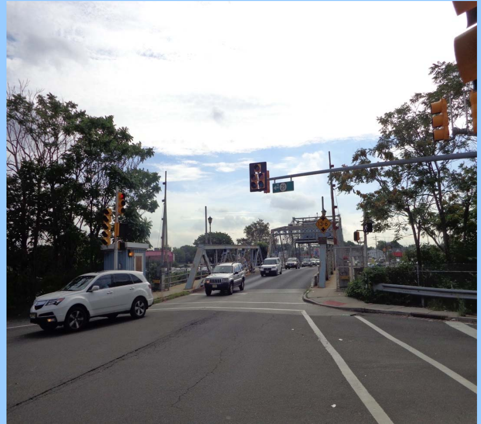
West approach to bridge at intersection with Route 21 ramps & Park Ave.
