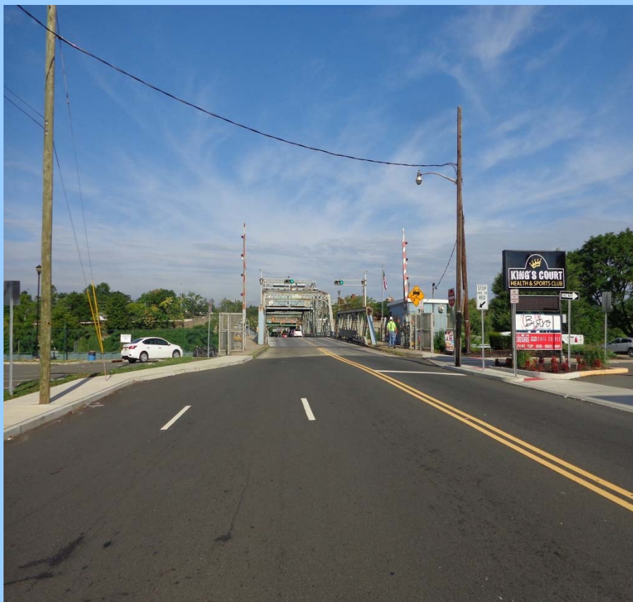
Bridge East Approach Roadway Looking West – Note no shoulders
