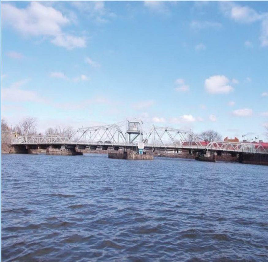
Bridge Navigation: 7-ft vertical clearance at MHW, 65-ft channel width
