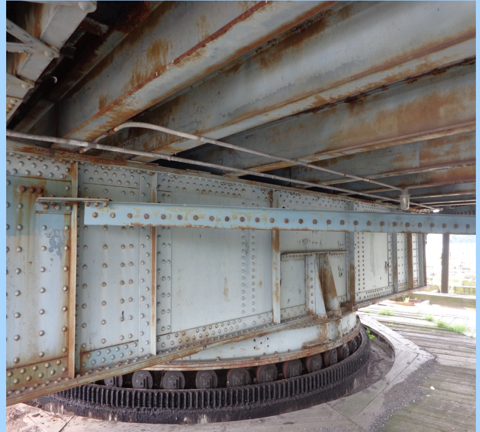
Swing Span Center Pivot
