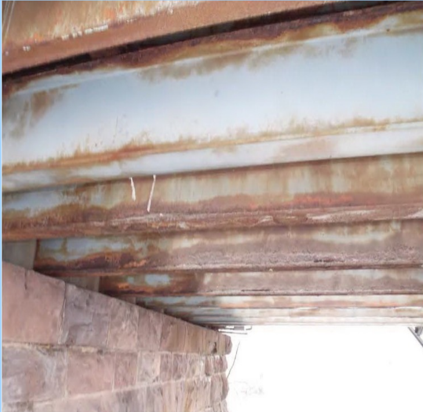
Severe corrosion of stringers in West Approach Span
