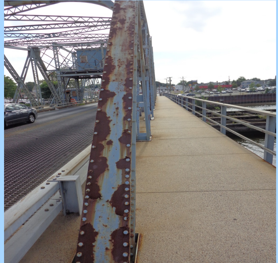
Corrosion of west approach pony truss span
