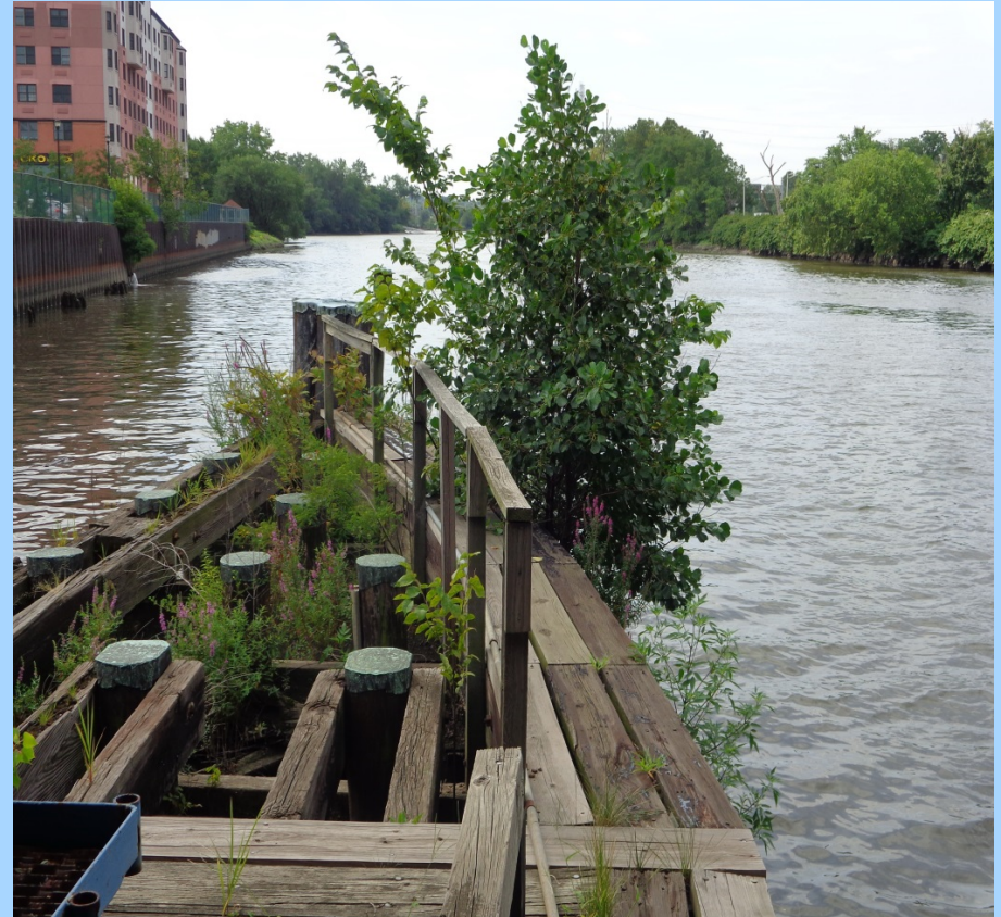
Advanced decay through pier fender system looking downstream
