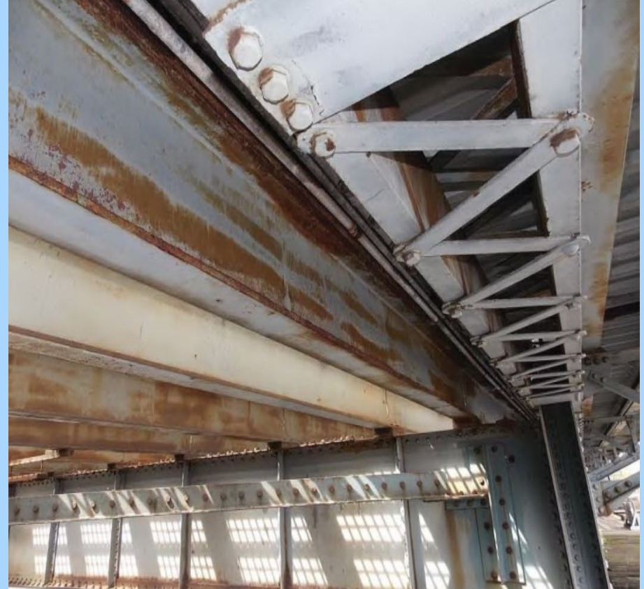
Moderate to heavy corrosion of stringers in swing span
