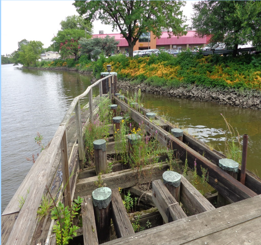
Advanced decay through center pier fender system looking upstream
