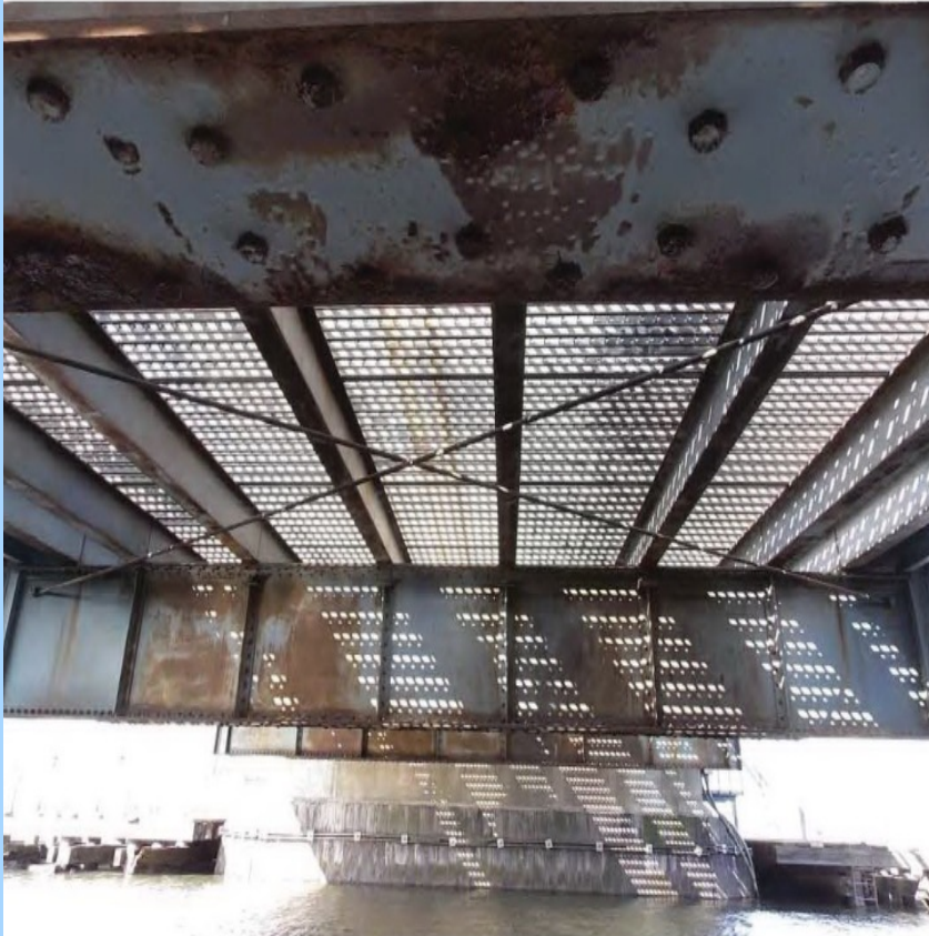
Floor beams & stringers of East Approach Span
