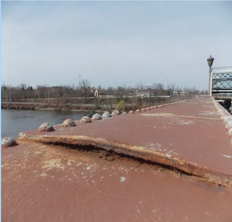
Severe corrosion of top of east approach pony truss & deterioration of rivets
