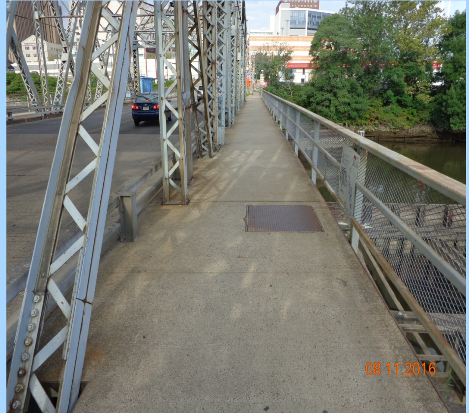
Substandard bridge railing (typical)
