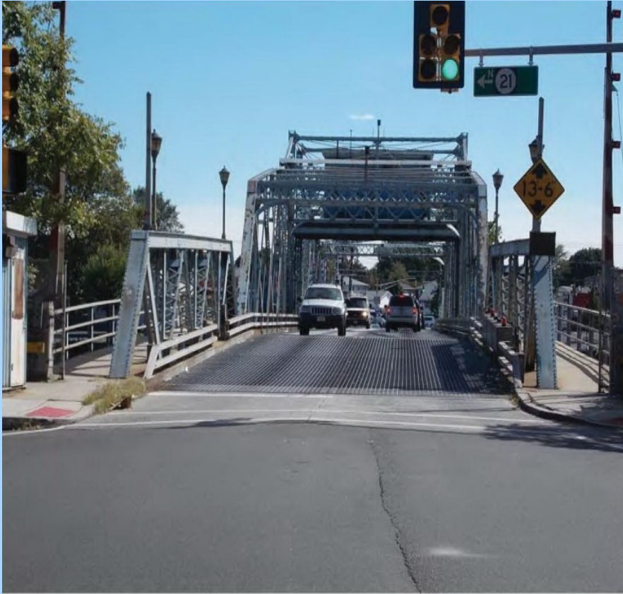
Substandard vertical clearance
