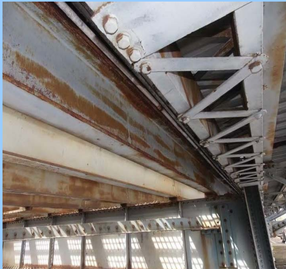
Moderate to heavy corrosion of stringers in swing span
