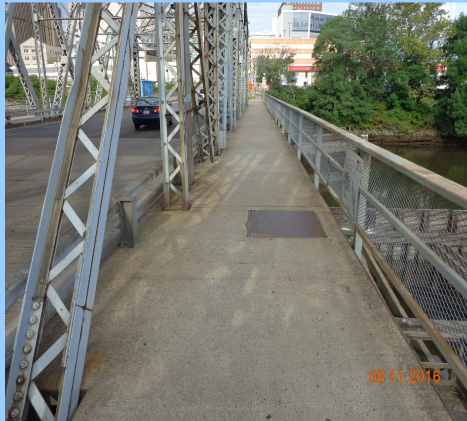
Substandard bridge railing (typical)
