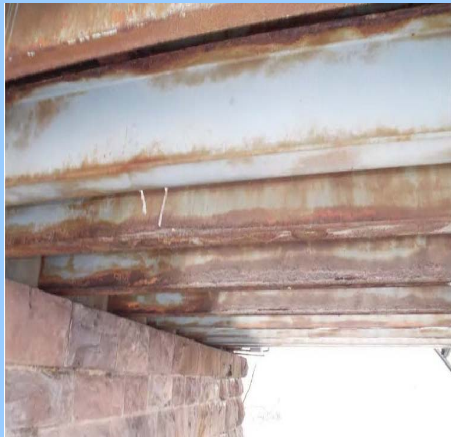
Severe corrosion of stringers in West Approach Span
