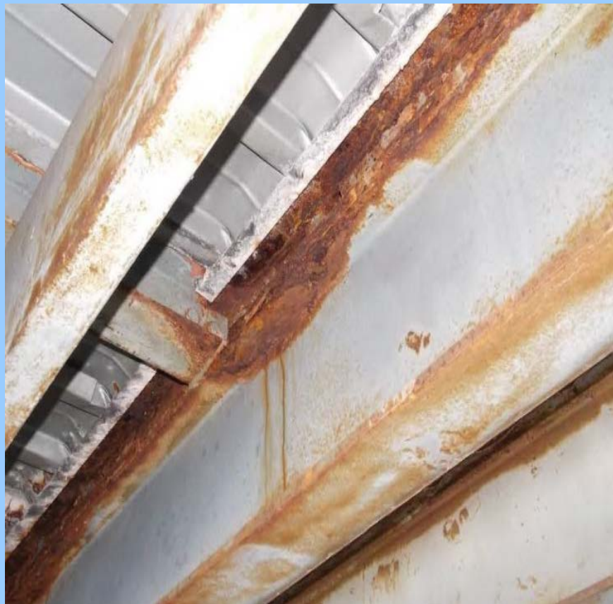
Severe corrosion in top flange of north curb line steel stringer
