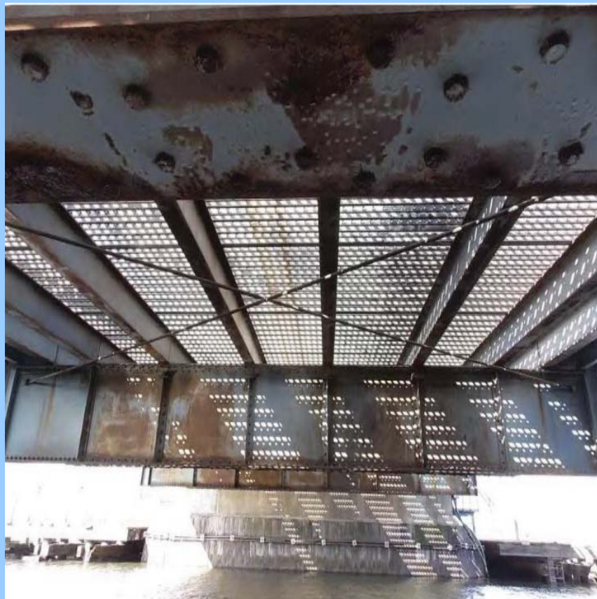
Floor beams & stringers of East Approach Span
