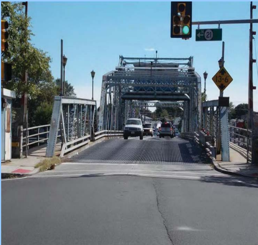
Substandard vertical clearance
