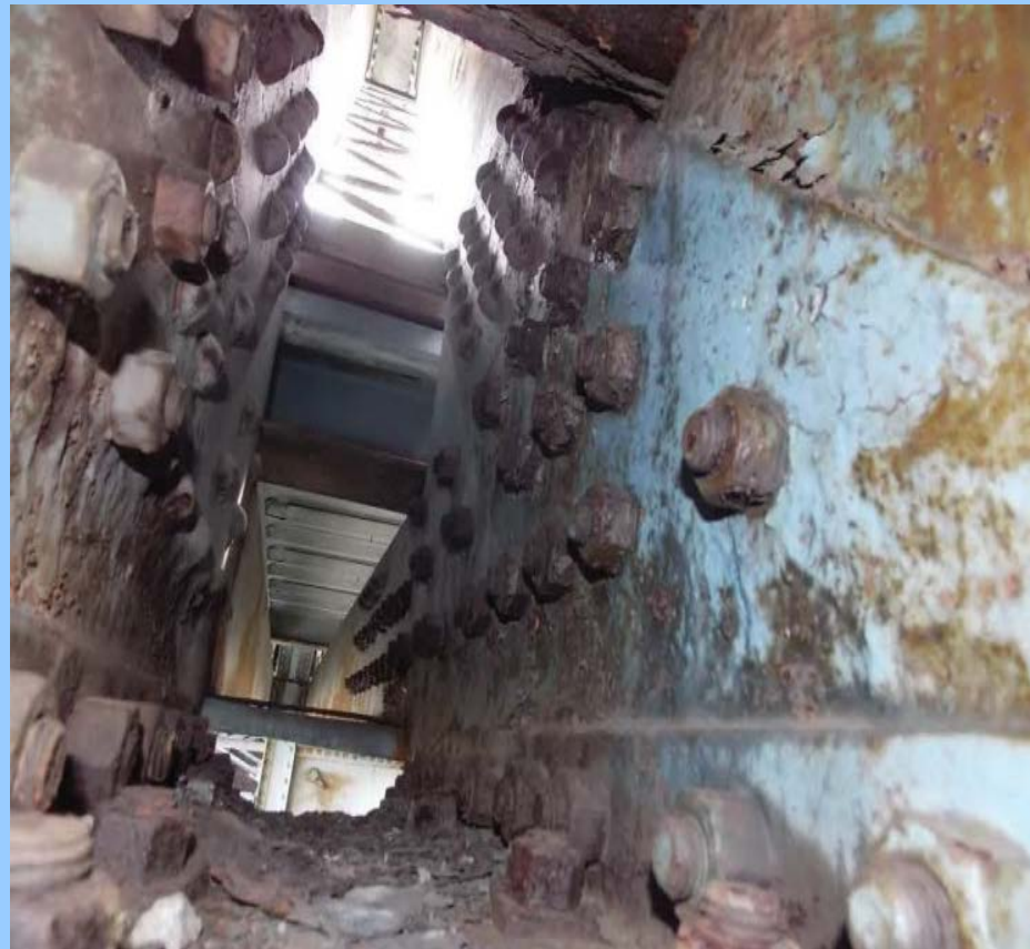
Section loss of gusset plate in East Approach Span
